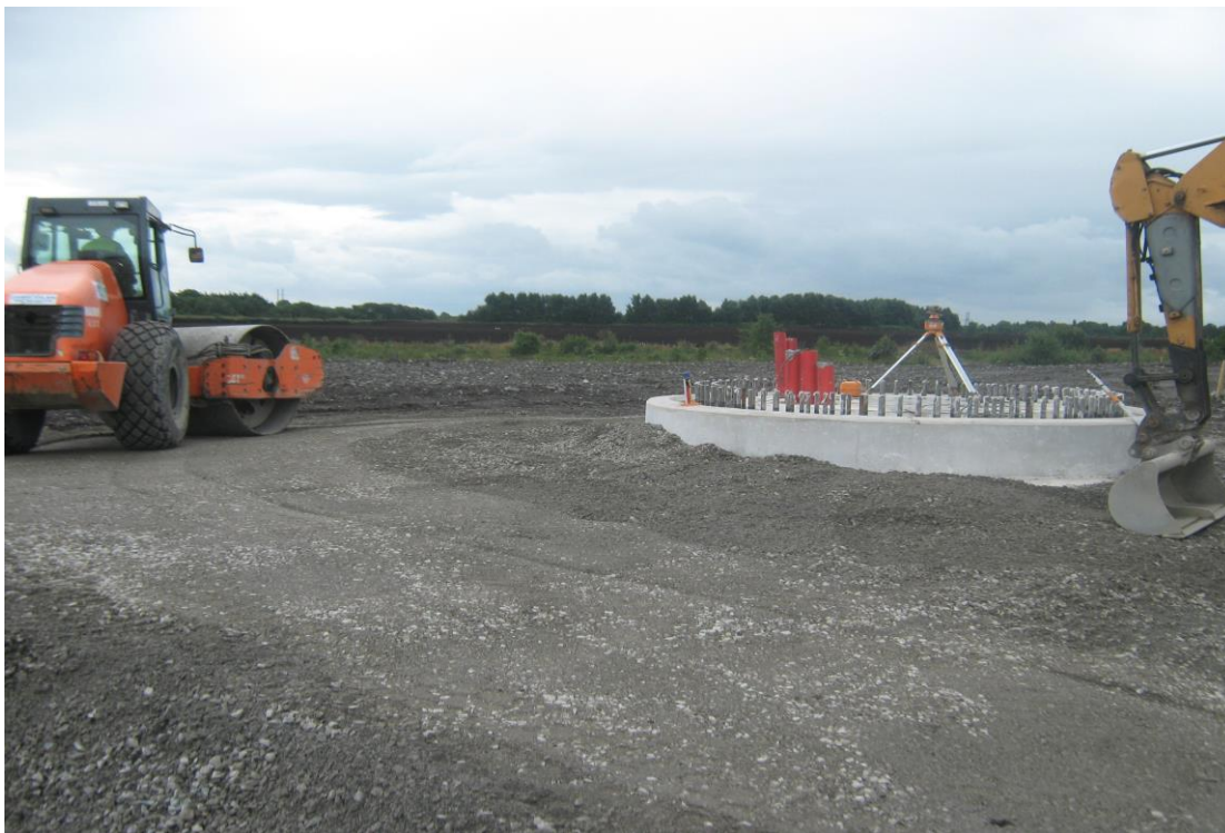
Compaction and backfilling of foundations.
