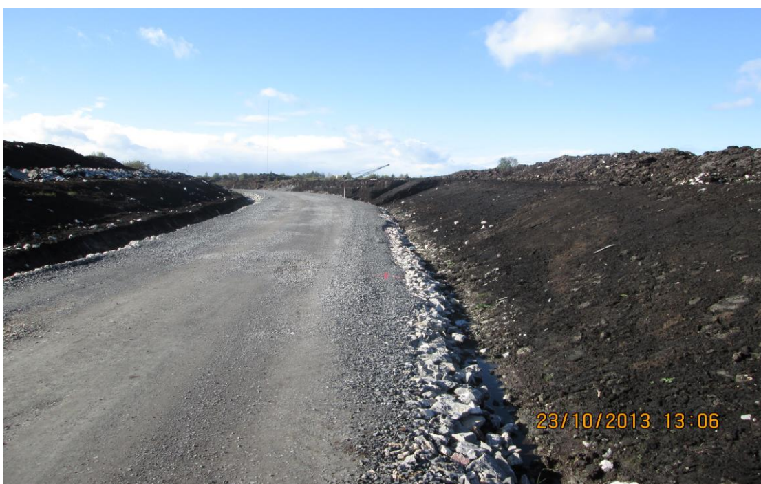
Road completion level at 804 formation level along with swales for drainage.
