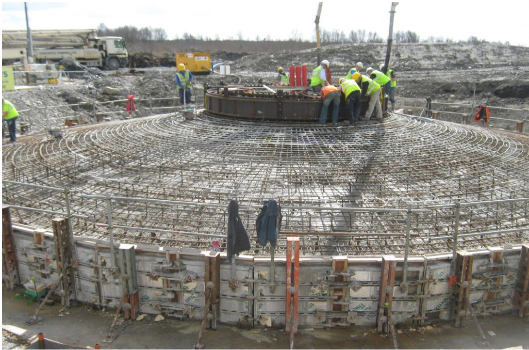
Typical concrete pour and formwork.
